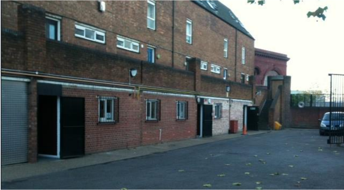
Image 1: View of office space (previous undercroft)
